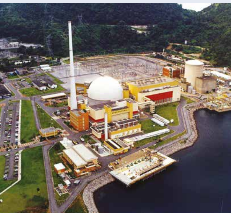
📍 The Angra Nuclear Power Plant, Angra dos Reis, Rio de Janeiro, Brazil. Two pressurized water reactors, Angra I, first connected to the power grid in 1985, and Angra II in 2000. A third reactor, Angra III, is due to enter into service in 2015.
